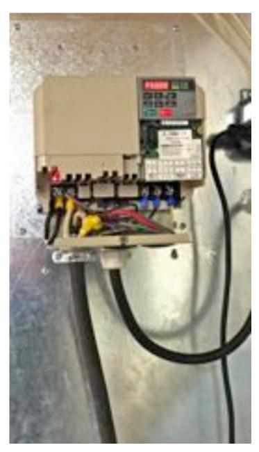
I could then bring in the two 220VAC single phase wires from the same line that had driven my Clearvue Cyclone unit and connect them to the input terminals on the VFD. These are the black and white wires on the left side of the VFD in this photo. The three three phase wires coming from the motor connected to the U1, V1 and W1 terminals on the output side of the VFD. These are shown as the three right most terminals in the photo.
