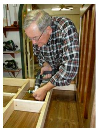
Once you also add the leaf guide pad assembly, use screws to pin these dovetails in place and you are nearly done. Notice how handy the Festool right angle attachment for the drill is in getting into the tight recesses of the frame.
